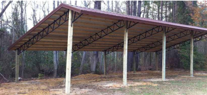
Pole structures. Photos from the internet by Panhandle construction companies.
