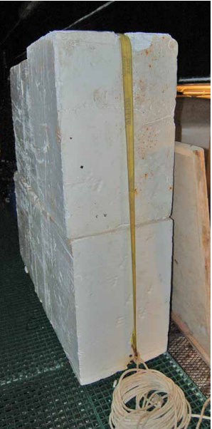
Substructure under tank: 2' foam blocks. Bottom row: Aquarist deck behind tank. Reference photos: Oklahoma Aquarium, Tulsa
