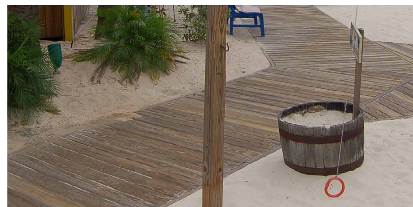
Below: Wood decking either level with the ground as shown below or 6" above the ground, to keep visitors on the path. Also consider a low rope railing.
